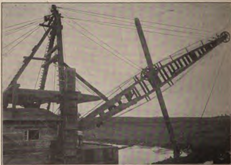
Boom and Dipper Handle of Floating Dipper Dredge.
